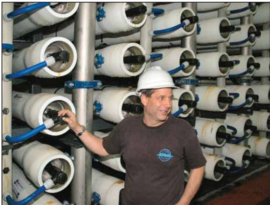
Micha Taubman, the operating manager of Israel's desalination plant at Ashkelon — the world's largest, most technologically advanced and economical — stands next to some of the 40,000 membrane units that are the heart of the purification technology.
